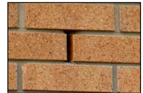
Open perpend can be uneven
