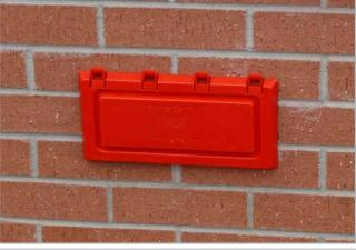
3) Your air brick is now protected Remove the cover as soon as flood water has receded
