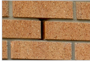
Open perpends can be uneven
